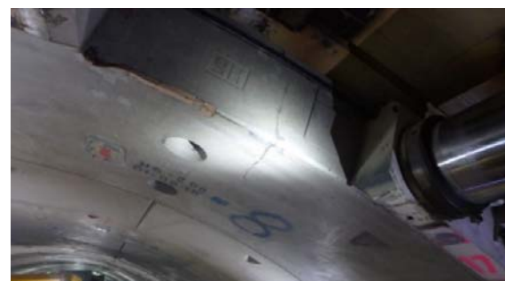
Figure 9. Cracks on segment (TTR1172)
