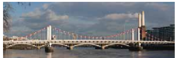
Chelsea Bridge-London UK - one of many monitored as part of the Thames Tideway project
