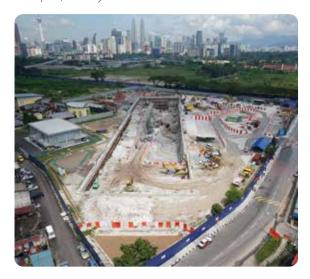
The KVMRT will be integrated with existing LRT, Monorail, KTM Komuter and bus network marking a new milestone in Malaysia's public transport system. The first phase of the project is the Sungai Buloh-Kajang Line (SBK) with a 9.3km underground alignment between Semantan North Portal to Maluri South Portal. This includes seven station boxes (25-45m deep), three emergency escape shafts and two intervention shafts.
